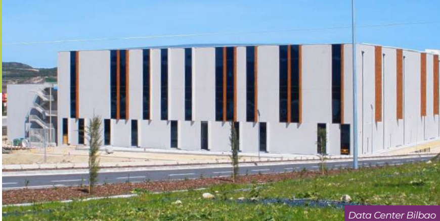
Data Center Bilbao
